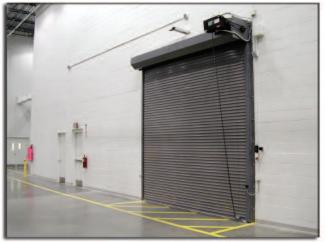
ADT Rolling Steel Fire Doors are designed to automatically close in case of fire and stop it from spreading from one area to another for a maximum of 3 hours. Doors up to 159 sq. ft. in area and up to 13'6" in width or 12'0" in height are manufactured with UL Labels Class A , B,or C. Doors over these dimensions but less than 30'0" wide and 24'0" high are supplied with UL oversize certificates. Although UL rated and automatically closing, they can still be used as coiling service doors.
